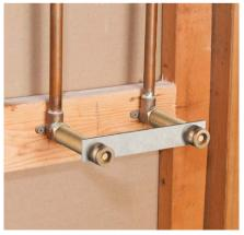
Hot/Cold Supply Lines Simple hot and cold water lines are the basis for installation.
